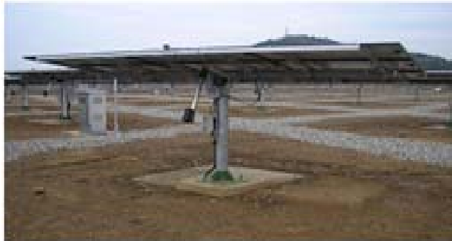
Fig. 3-3 One directional tracking PV array
