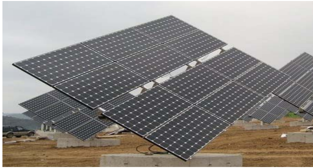
Fig. 3-4 Bidirectional tracking PV array
