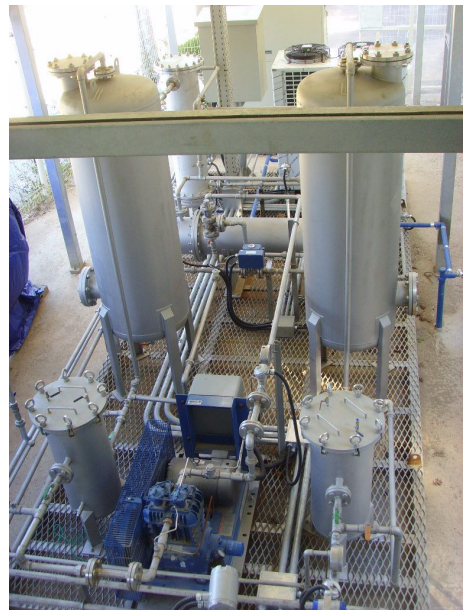
Figure 5. LFG Cleaning/Pretreatment System for Microturbine
