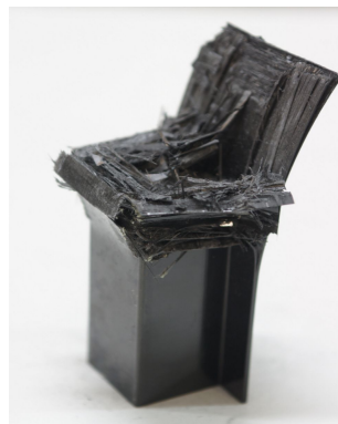
Photo. 17 Collapsed shape of CFRP hat-shaped sectional member, 3 interface (wet specimen, outer angle 90^\circ )
