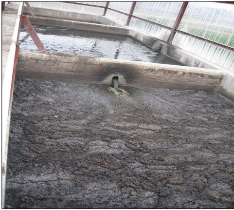
(A) Before stabilization.
