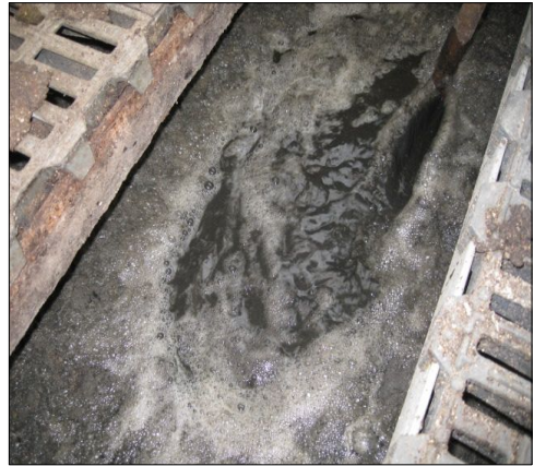
(B) condition of slurry pit.
