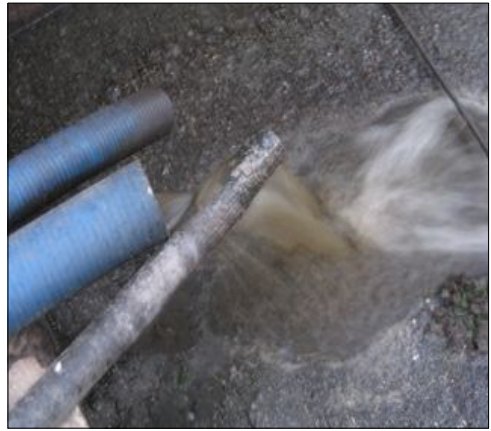
(B) After stabilization.
