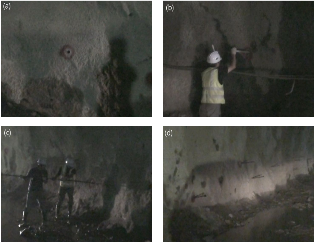
Figure 4.2 Installation process of rock and spiral bolts in a borehole; (a) Borehole, (b) Injection of resin, (c) Insertion of rock and spiral bolts, (d) Completion of installation
