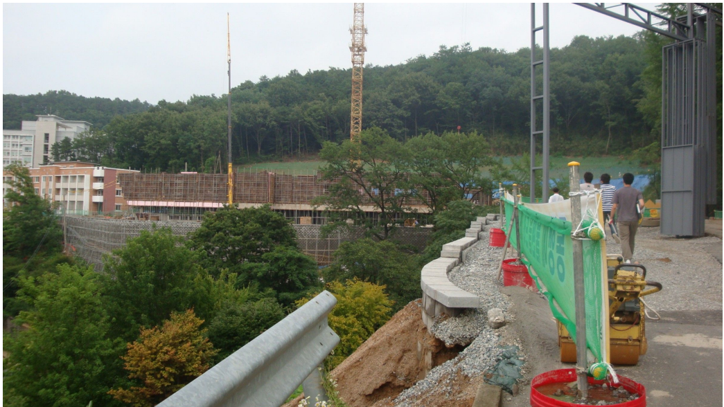
Figure 4.11 Photograph of construction site.
