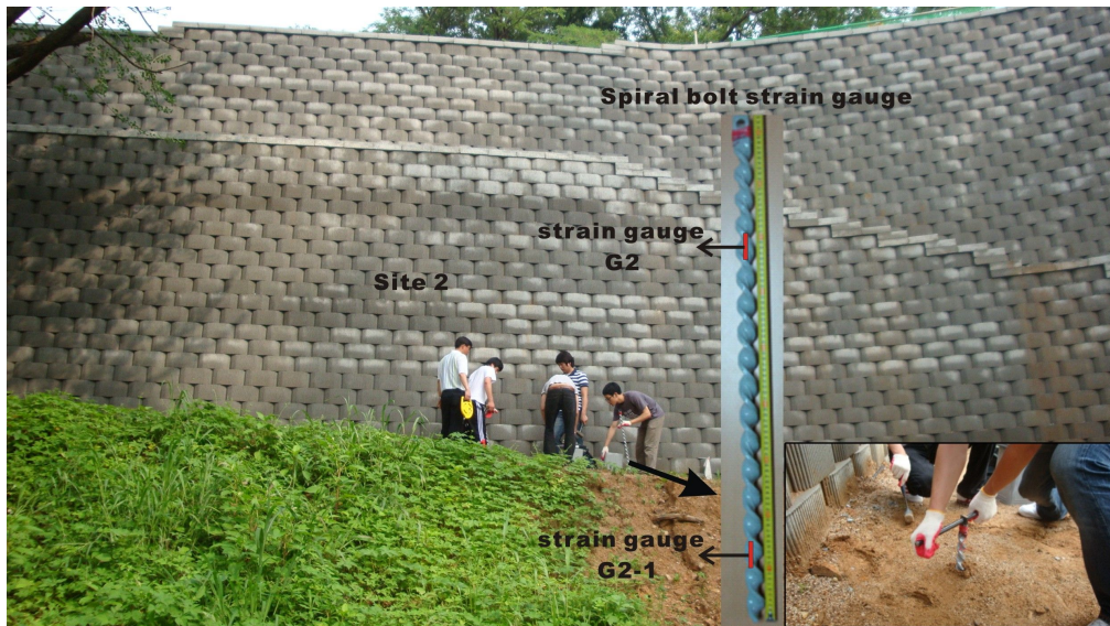
Figure 4.15 Photograph of spiral bolt stain gauge installed on Site B.
