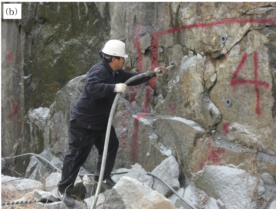
Figure 6.3 Process for in-situ pull-out test: (a) Boreholes for pull-out test, (b) injection of cement-mortar, (c) installation of test equipment, (d) in-situ pull-out test.
