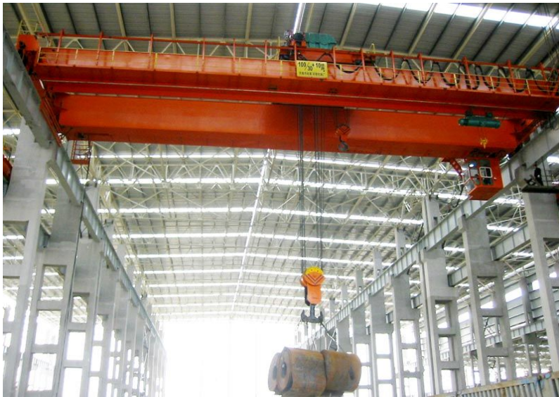
Fig. 1-1 Bridge crane(Henan yuntian company)
