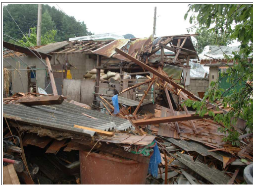
Fig. 50. Farm house damaged by gust.
