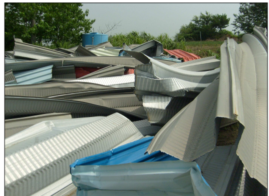
Fig. 4. A factory roof is damaged by gust(Surogli Baksan Gimjae city).
