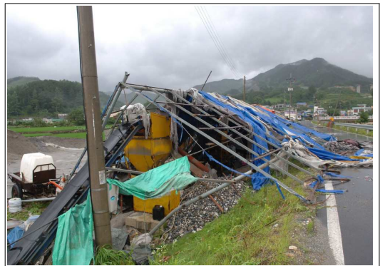
Fig. 51. Vinyl house damaged by gust.
