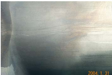
(c) Convex crack (MS7001FA +e 1st stage bucket)
