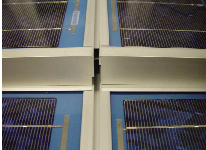
Fig. 4-4 Picture of horizontal joints
