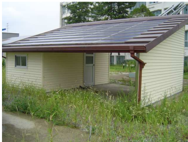
Fig. 4-6 Roof-integrated PV system model-house
