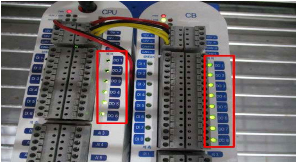
Fig. 3-129 Check DO LED lighting before test
