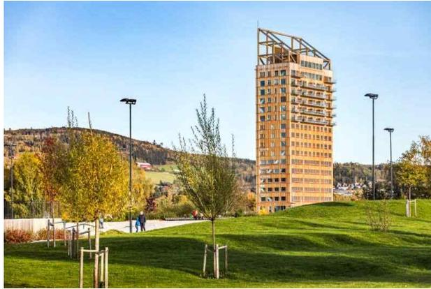
Figure 1.2 Mjøstårnet wooden building<sup>[5]</sup>
