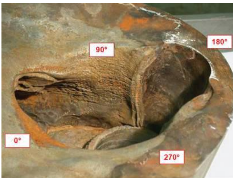
Fig. 1.14 Damaged CRDM area in David-Besse RPV[51]
