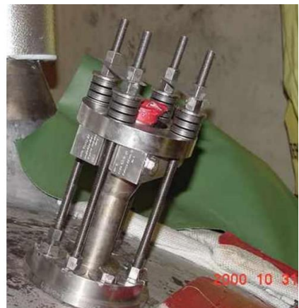
Fig. 1.24 Schematic representation of MNSA and installed MNSA[74]
