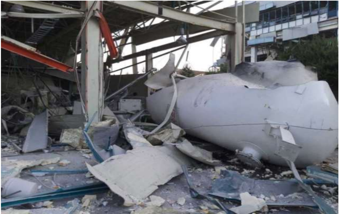
A) Gangneung Techno Park Hydrogen Storage Tank Explosion Accident [9]
