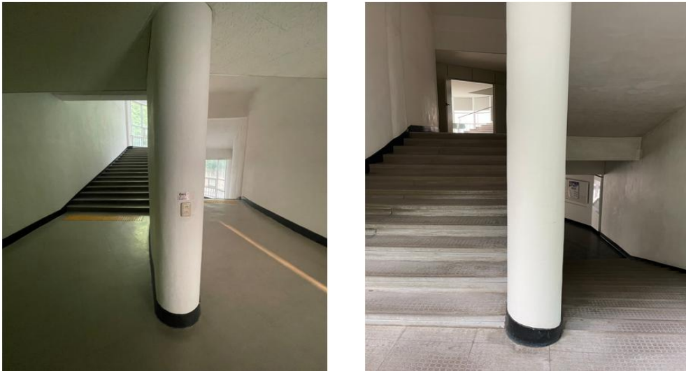
Figure 3.9. Closed six-story staircase
