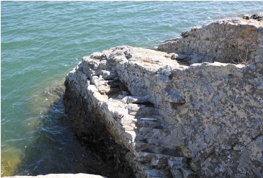
Fig. 35. Cross section of columnar joint exposed after fracture by structural joint.
