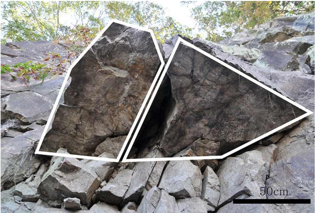
Fig. 52. Cross section of columnar joint across from Yongampo(port)(Site 2-B).
