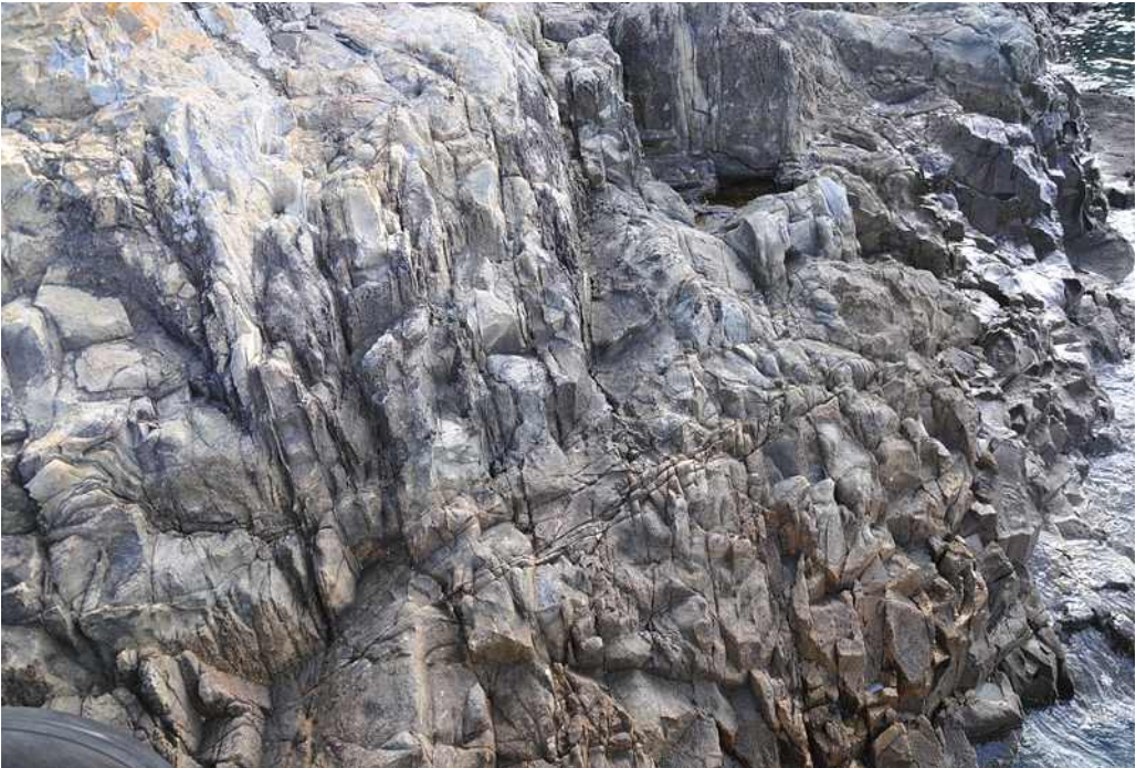
Fig. 25. Structural joint intersecting in the shape of an X(northern area).
