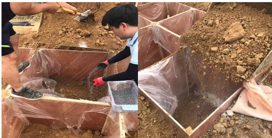
Fig. 4. Application process for S/S technology
