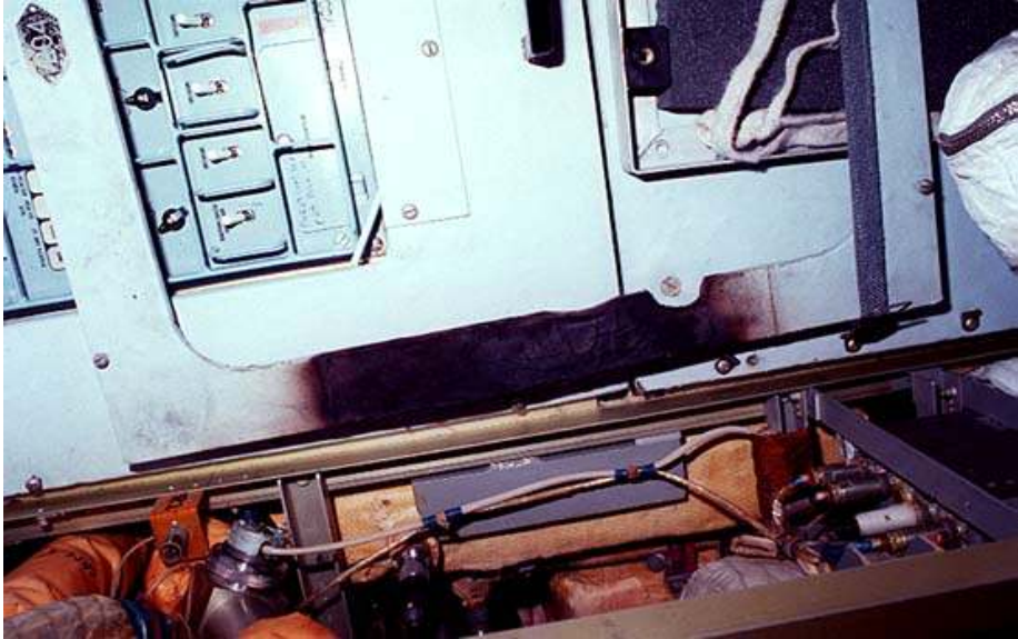
Figure 1.4 Damages due to an Accidental Fire on Mir Space Station [6]
