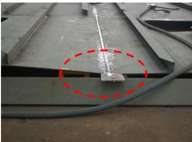
Fig. 1.1 Welding distortion in ship-yard
