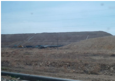
Erosion of waste rock
