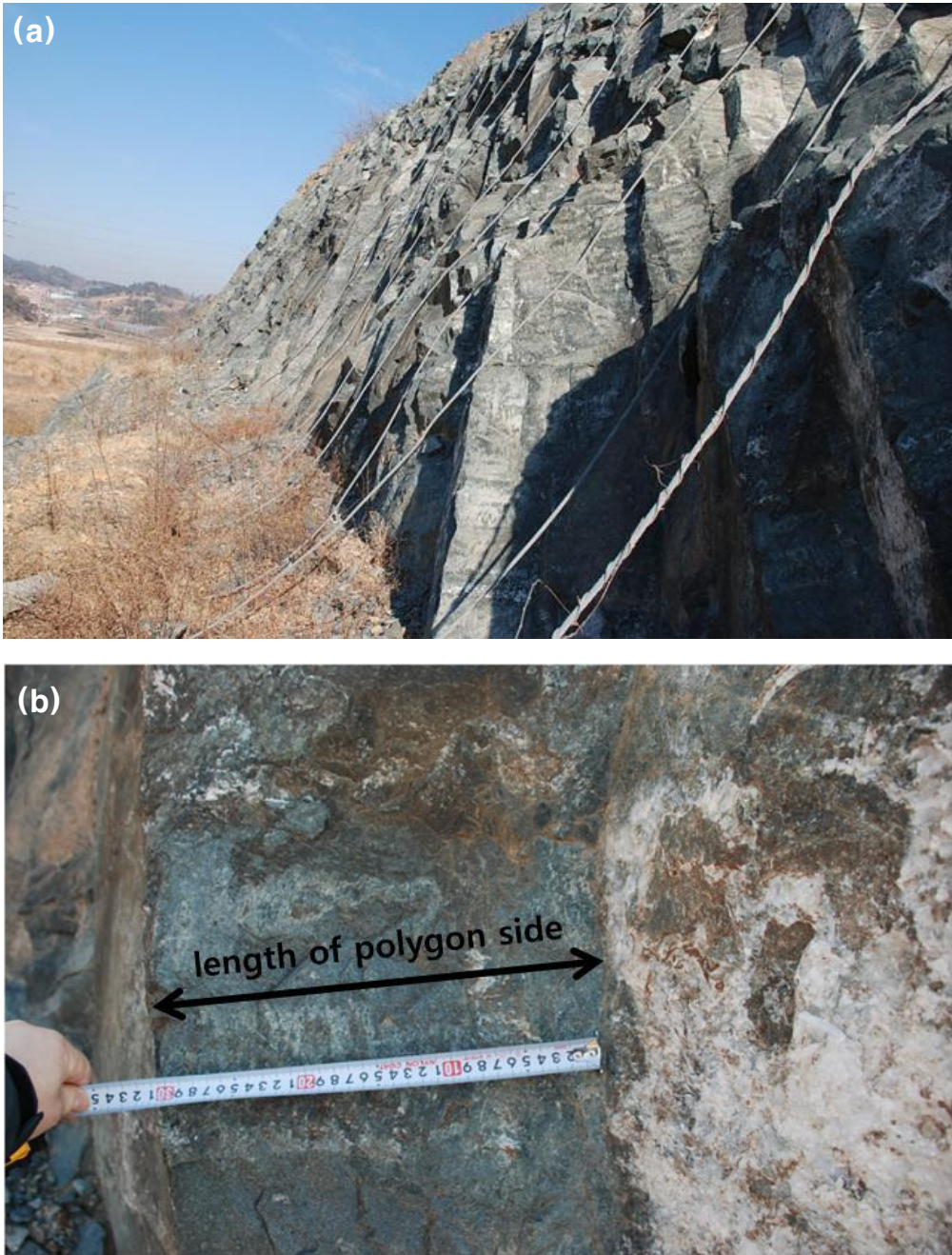
Fig. 29. Photographs of Suncheon area(SC-5).
