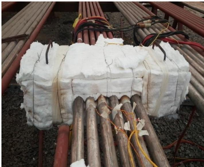
Fig.6 General PWHT of Tube Condition for 30min
