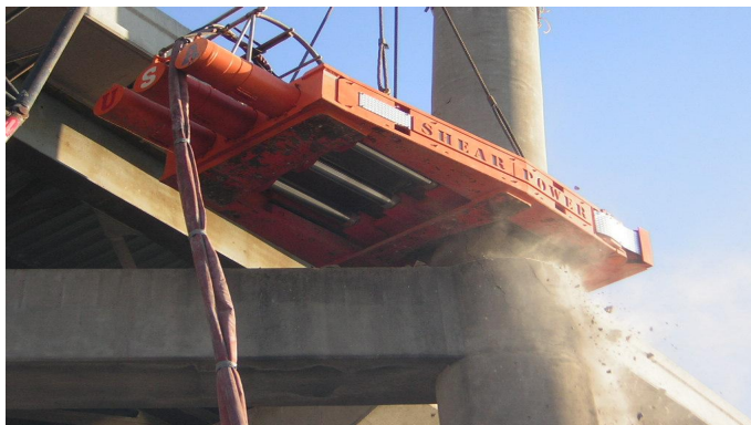
Fig 15. Shear Cutting
