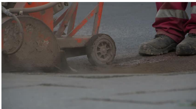
Fig 12. Mechanical Saw Cutting
