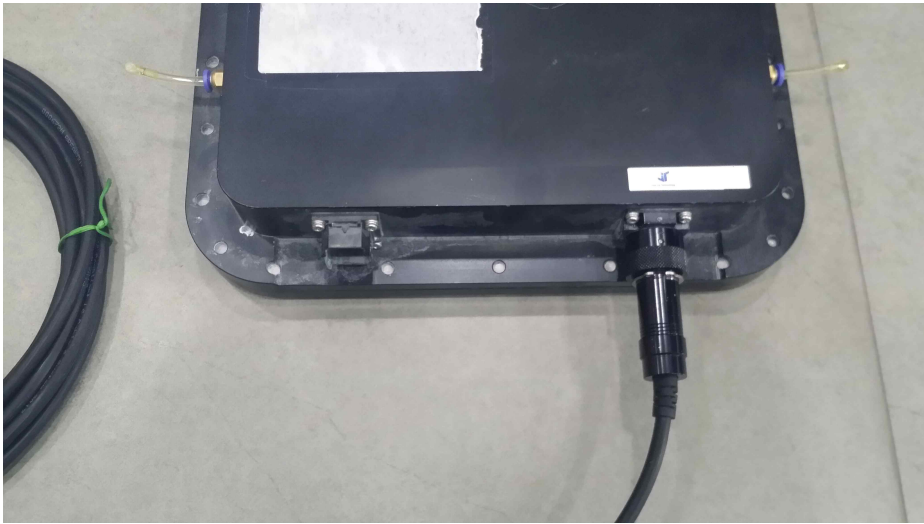
Fig. 3-24 Image of Air-leakage test
