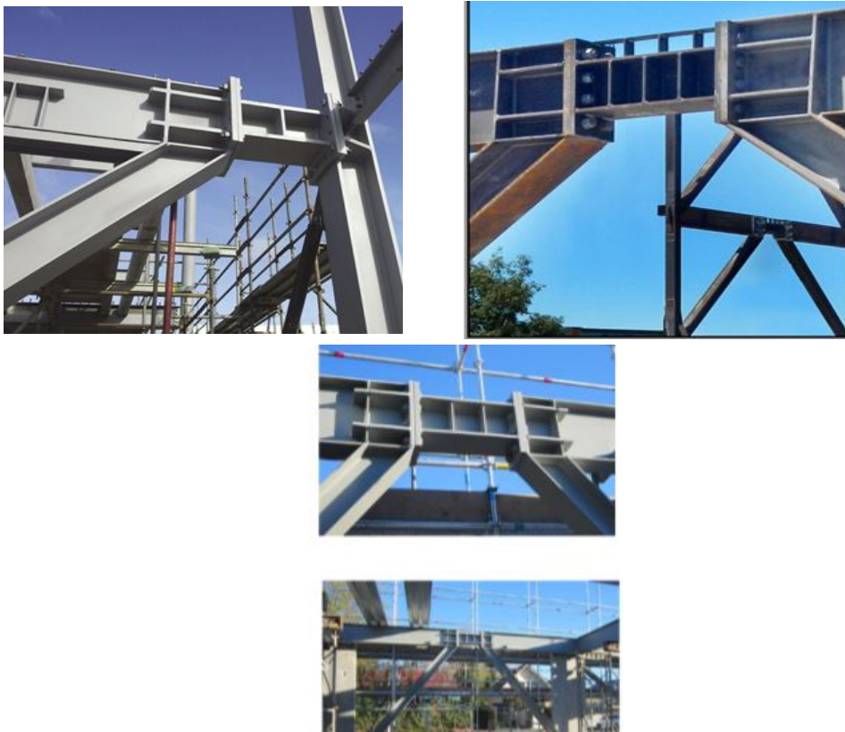
Fig 1.4 New Zealand Examples of EBFs with Removable Links [1]
