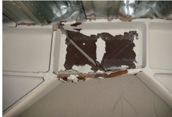
(a) Fractured EBF active link in Pacific Tower. (Image Spiire New Zealand Ltd.)
