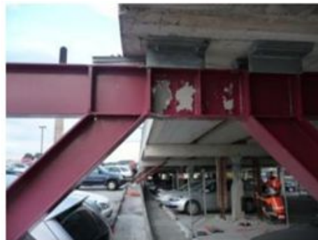
(c) Fractured link at lower level EBF
