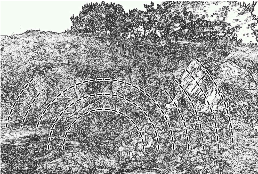
Fig. 117. Photograph and sketch of columnar joint structure in Guryongpo. (dot line: isothermal lines)
