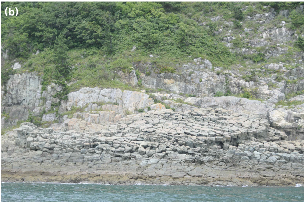
Fig. 79. Photographs of columnar joint in NH-03(a), NH-05(b).
