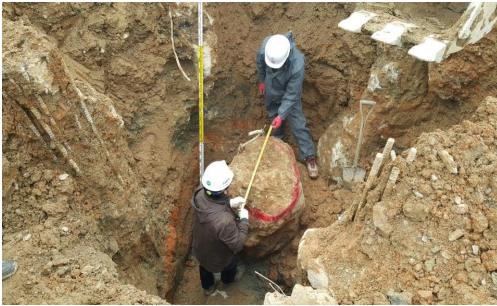
Figure 4.31 Excavation of C.P.R bulb
