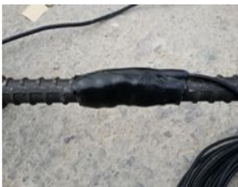
Figure 3.13 The secondary Waterproof processing
