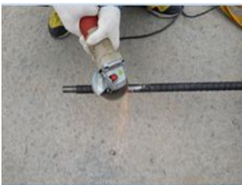
Figure 3.10 Processing of sensor installing surface
