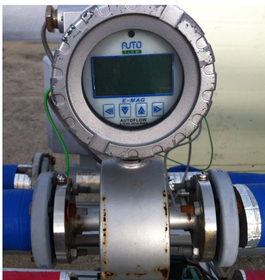
Fig. 2.4 Photograph of flowmeter
