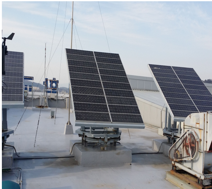
Fig. 26 The installation of semi-fixed 3kW PV system
