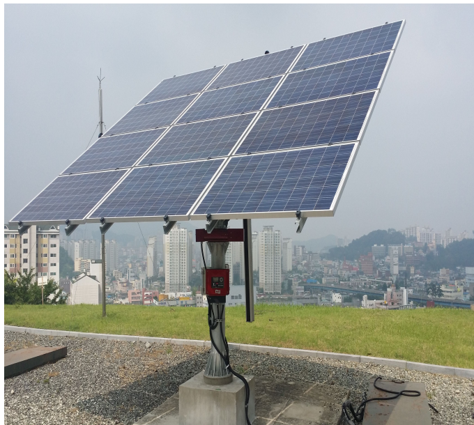
Fig. 10 The photo of tracking array
