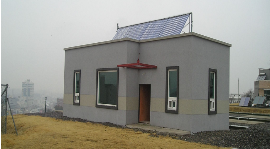
(a) Evacuated tubular solar collector installed insulation house
